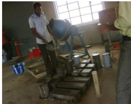
Fig 5.7 Placing of Fresh Concrete
