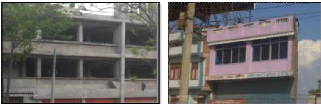
Fig. 1 Partially infilled frames
