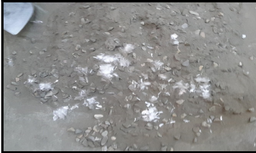
Figure 2. Addition of PPL fibers in concrete mix before addition of water
