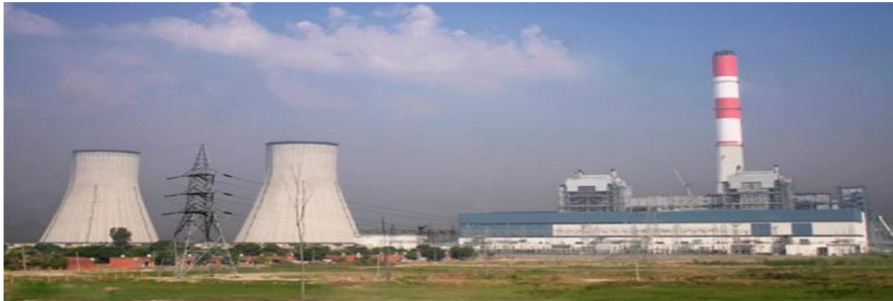
Fig 1. Photographic view of panipat thermal power plant
