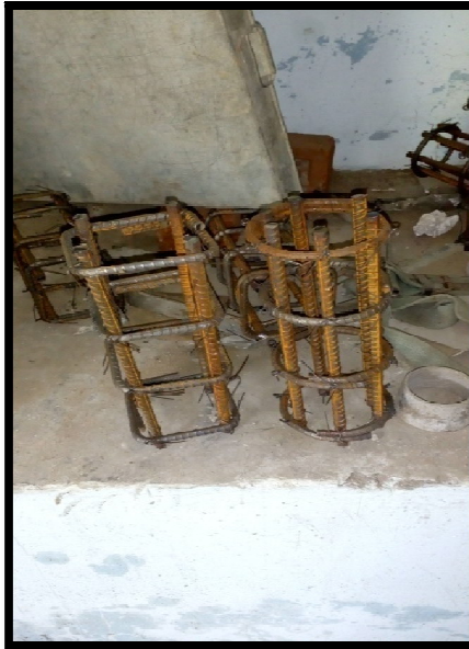
Fig.1 – detail of reinforcement
