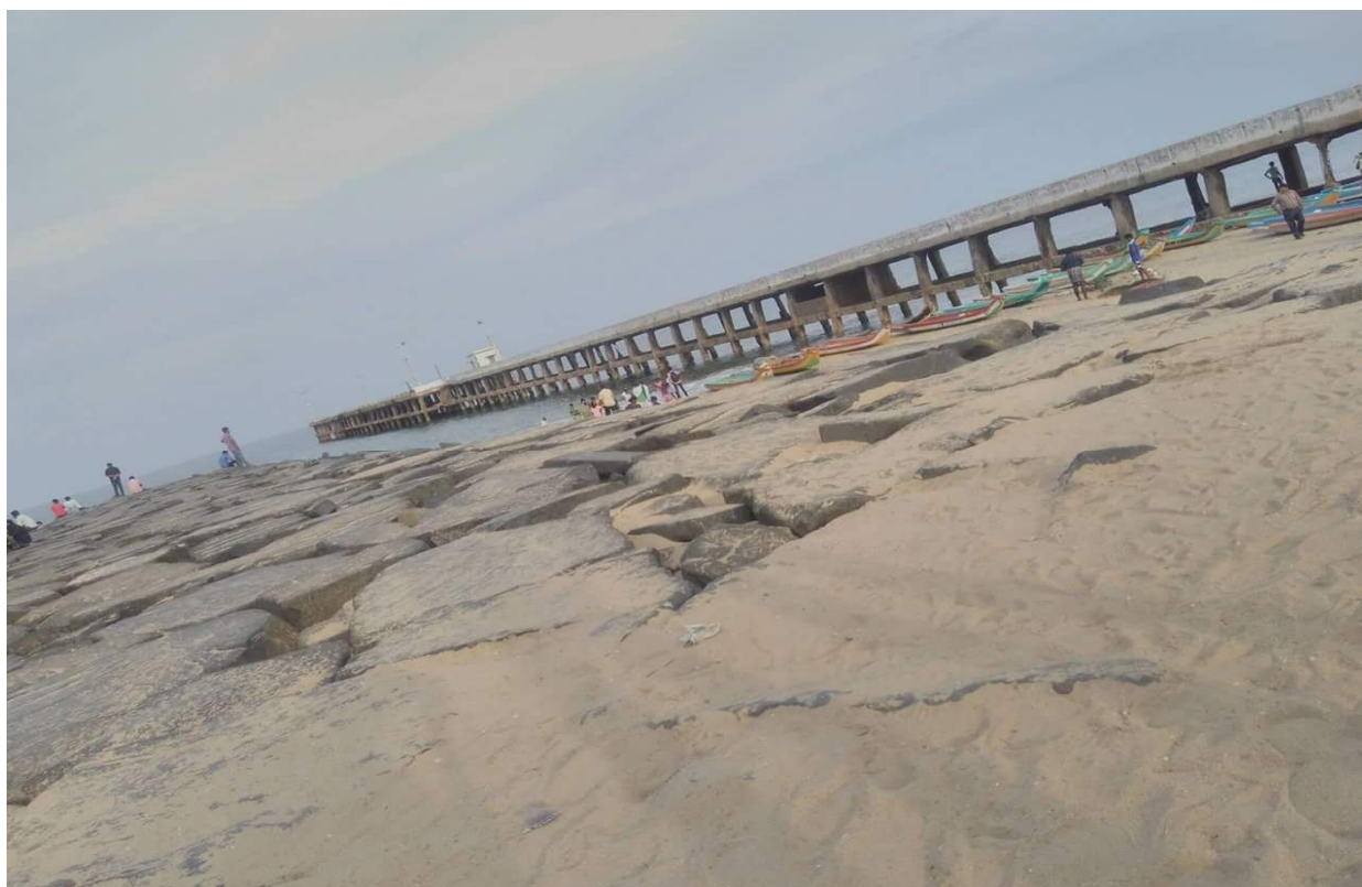
Fig 5. New pier at Pondicherry
