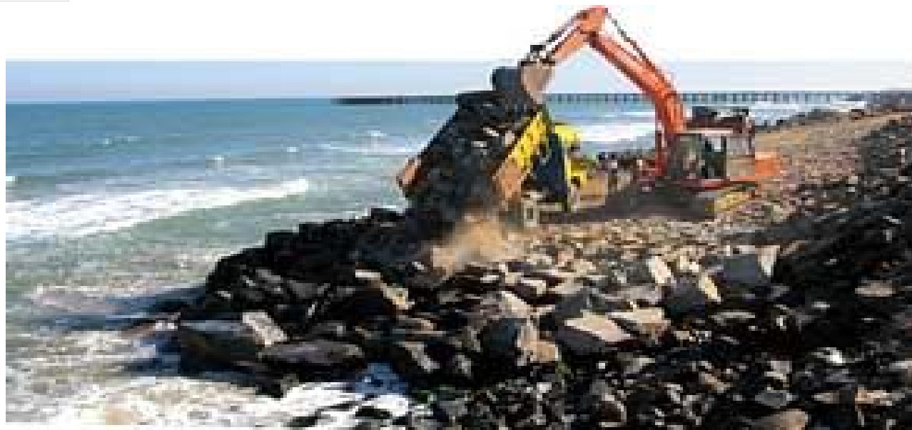
Figure 6: Rubbled Mound Construction At Puducherry Sandy Beach
