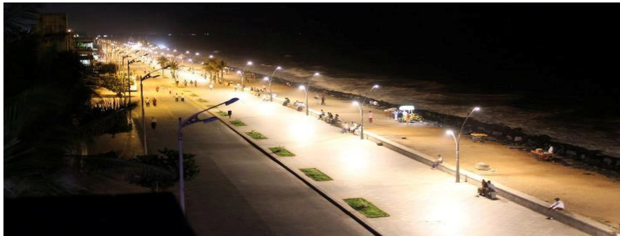
Fig 9 : Rubbled Mound seawall with walk way -2006
