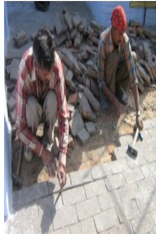
Removal of finishing brick
