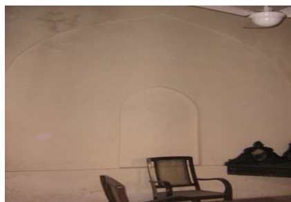
Restored lime plaster
