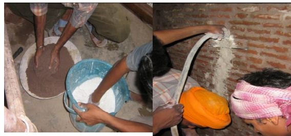
Lime grouting mixture
