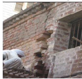
Crack in masonry
