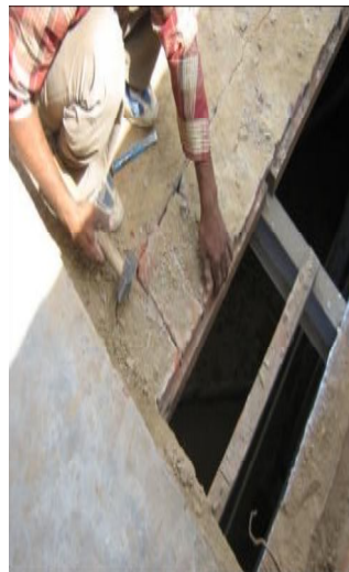
Removal of finishing brick
