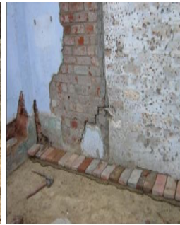
Brick tile on mud mortar
