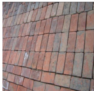
Finished brick tile layer
