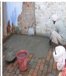
Neat cement slurry
