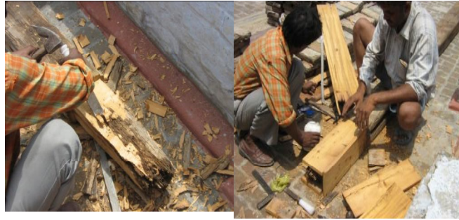
Removal of wood end
