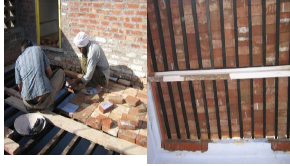
First layer of tile laid
