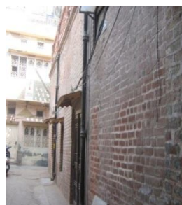
Restored Lime pointing
