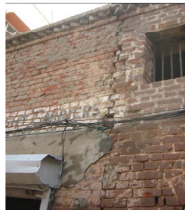
Crack in masonry
