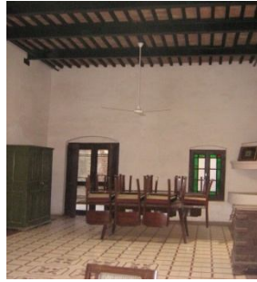
Restored roof & flooring
