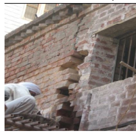
Crack in masonry
