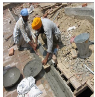
Casting of drainage
