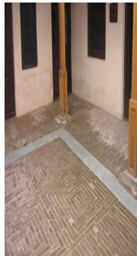
Brick on edge plinth protection in dry lime
