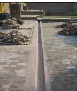
Finished drainage at terrace
