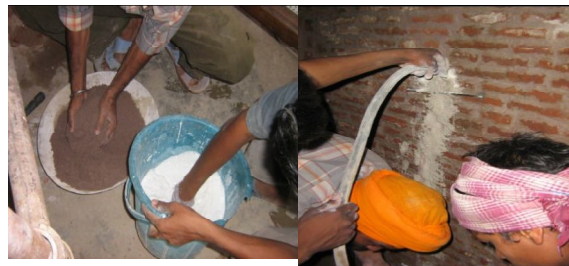
Lime grouting mixture
