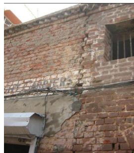
Crack in masonry
