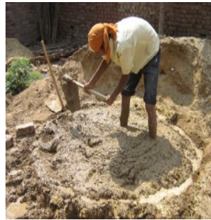
Mud mortar preparation
