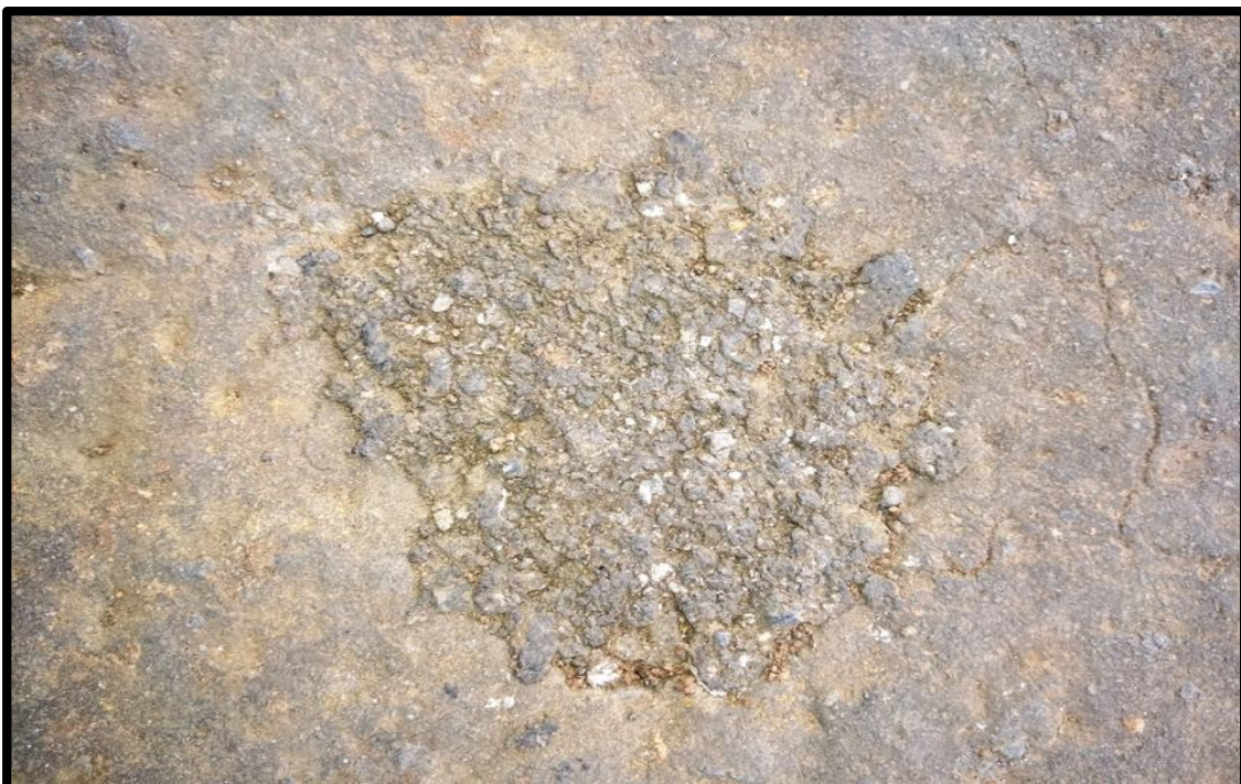
Fig.3 Pot Hole Repaired using WPA-Bitumen Mix.
