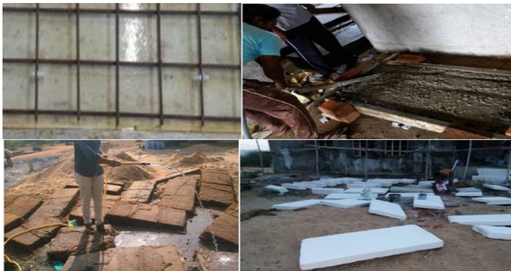
Fig 1: Photos showing the steps of one way slab casting until curing
