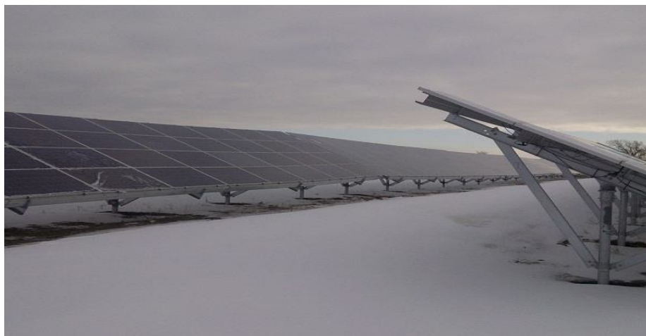
Figure 7. Typical row of solar panels in winter showing very little to no snow accumulation around foundation piles.
