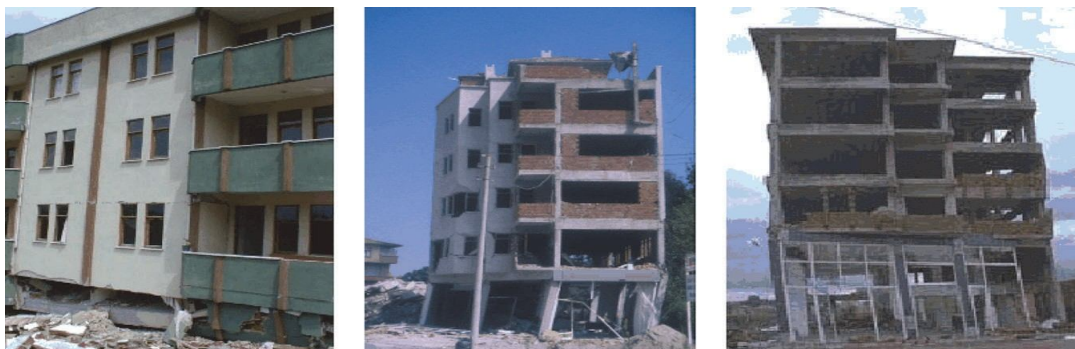
Figure 3. Damage to soft storeys
