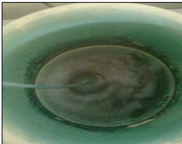
Fig-4 Aeration in SBR reactor.
