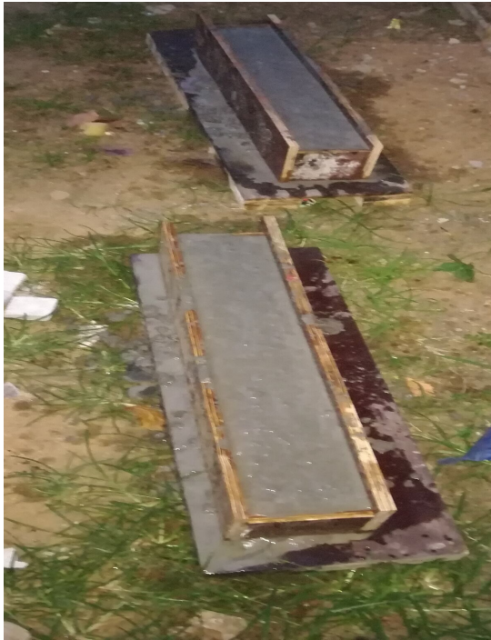
Fig2: Casted Columns
