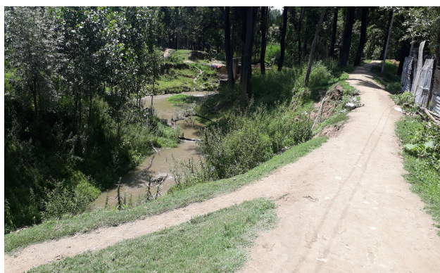
Fig.1: Existing embankment along the bank of river.
