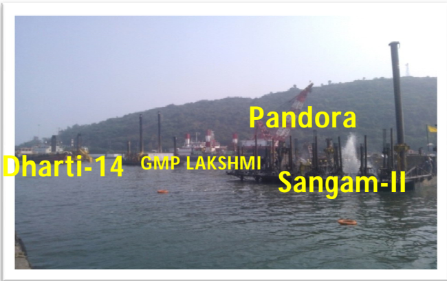
Fig 4.6 Dredging & Drilling/Blasting is in progress Block-F
