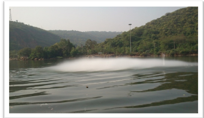
Figure 4.7 View of Blasting by Drill Barge 'SaiHaritha'
