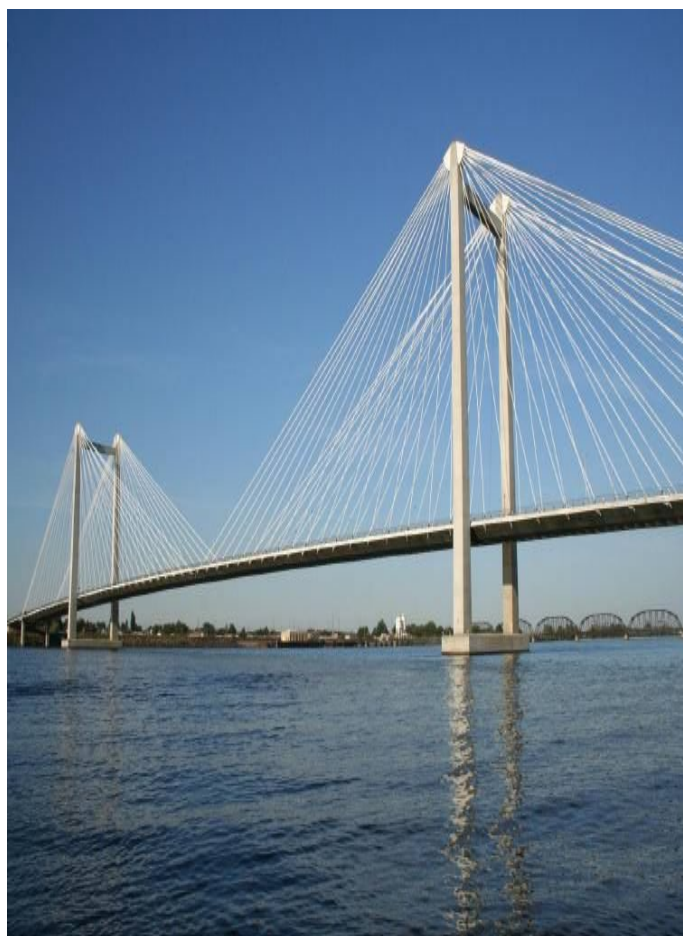
Fig-2: Cable stayed Bridge
