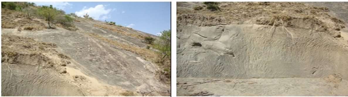
Fig. 1: Location of samples collection (at Powerhouse, UJH Multipurpose Project, J&K)
