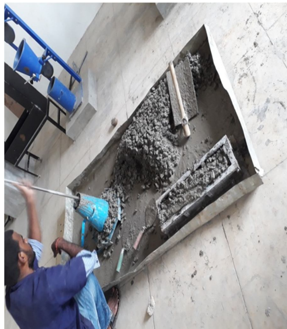
Fig. 9. Slump Cone Test
