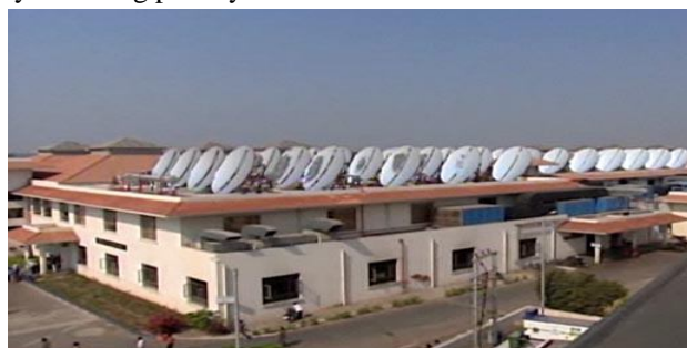
Fig.4.2 solar cooking system
