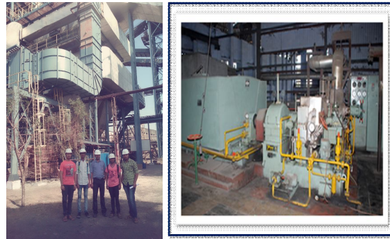
Fig.4.1 steam turbine at factory
