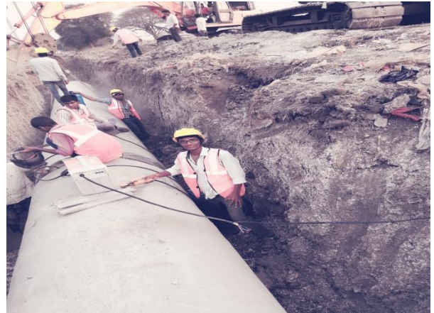
Fig 2:- New DI K7 Proposed pipes for construction
