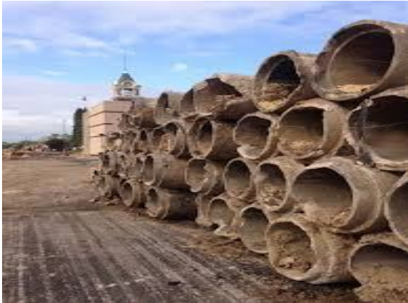
Fig 1:-deteriorated pipes removed from the existing system
