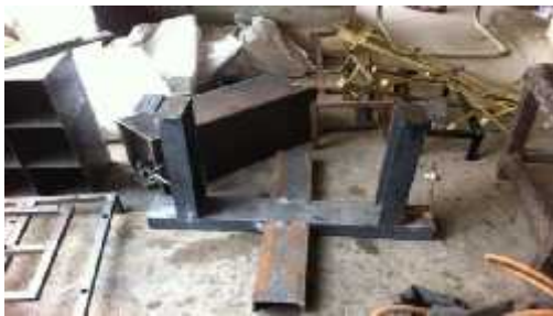
Fig.2 Fabrication of base stand
