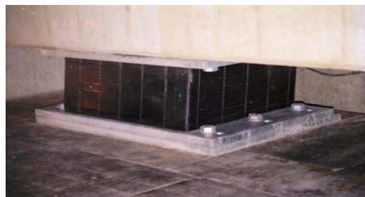
Fig. 6 High damping rubber bearing used in bridge
