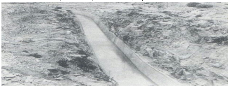
Fig 2. Cement Concrete Canal Lining
