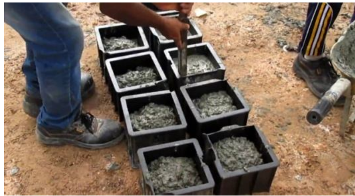
Fig: casting of cubes
