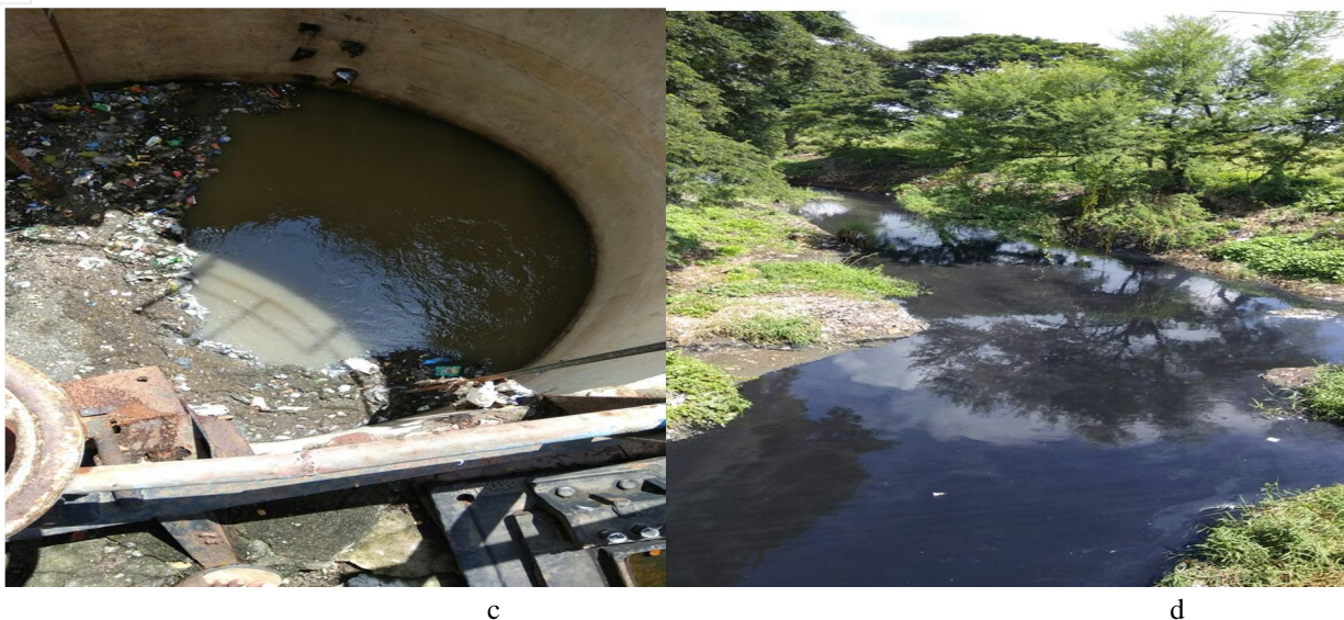
Fig.3. (a, b, c, d) Sewage treatment plant and Kala Nala
