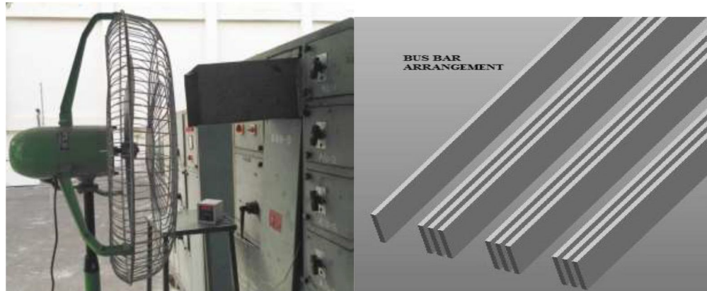
Figure 3 Experimental arrangement and Bus bar with 3 conductors per phase
