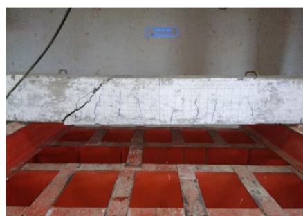
Figure 10 Crack Pattern after Loading
