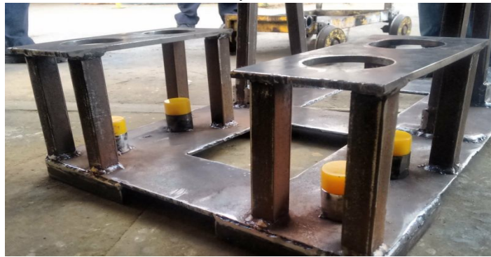
Fig No 5 Pinion box welding
