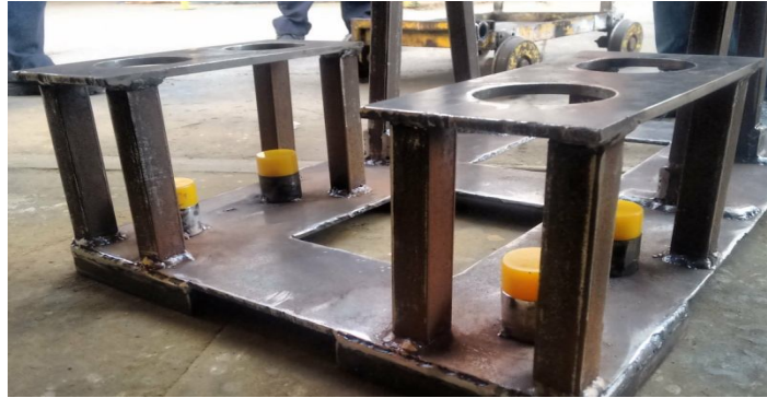
Fig No 5 Pinion box welding
