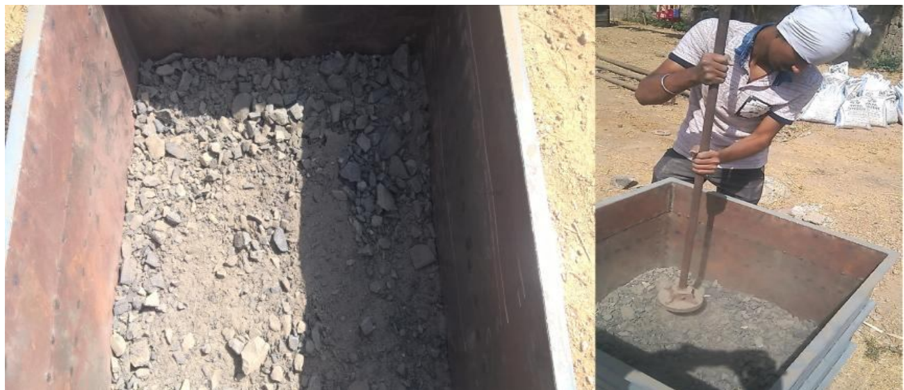
Figure 5 Laying and Compaction of Subbase
