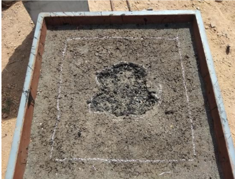
Figure 13 Position of Pothole
