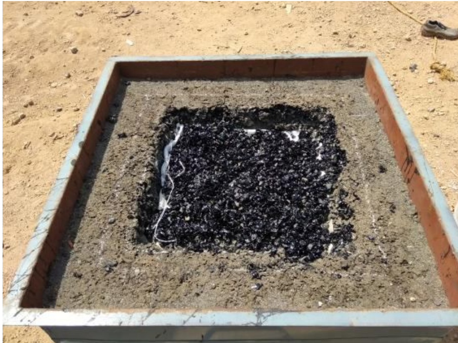
Figure 15 Laying of Bitumen Concrete
