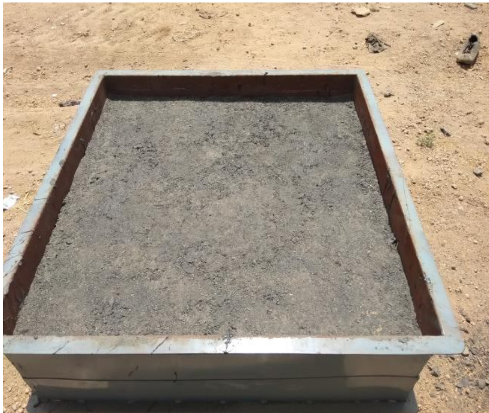
Figure 10 After Completion of Laying and Compaction of Wearing Course
