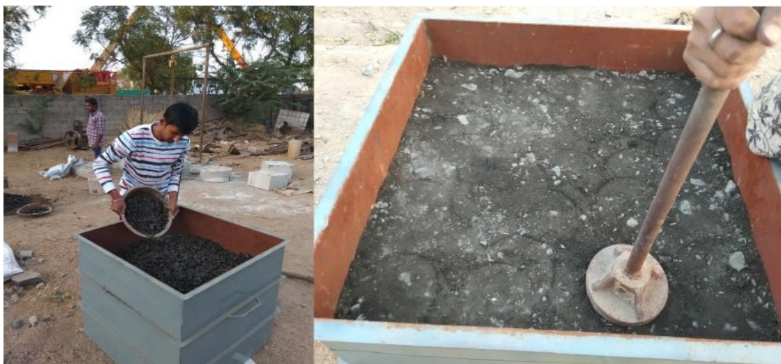
Figure 8 Laying and Compaction of Base course/WMM
