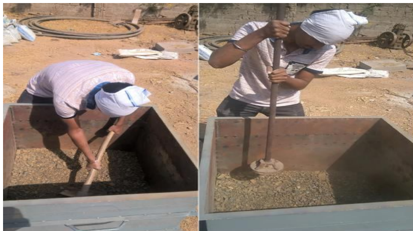
Figure 4 Laying and Compaction of Subgrade
