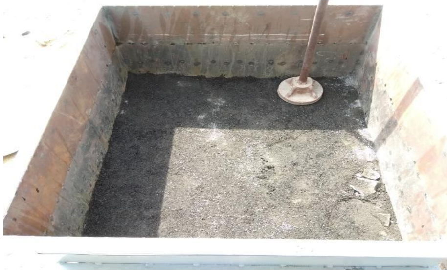
Figure 6 Laying and Compaction of WBM
