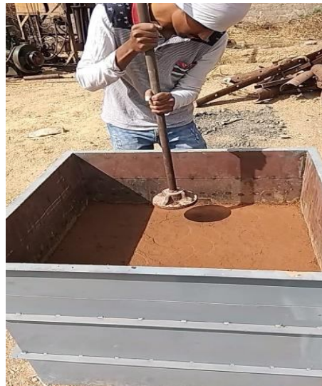
Figure 7 Laying and Compaction of WBM final layer
