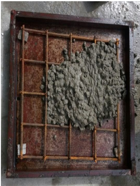
Figure 2: Slab mould with reinforcement
