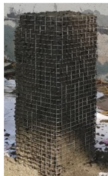
Fig. 2 ferrocement jacketing
