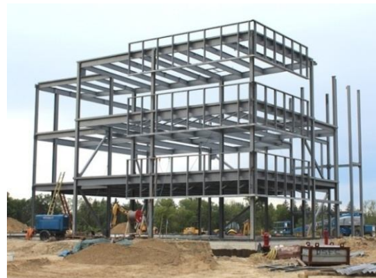
Fig. 2: Steel Frame structure
