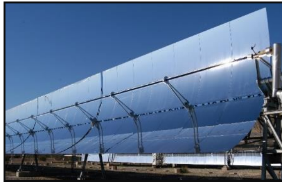
(Fig. No. 5.1 Parabolic Trough)
