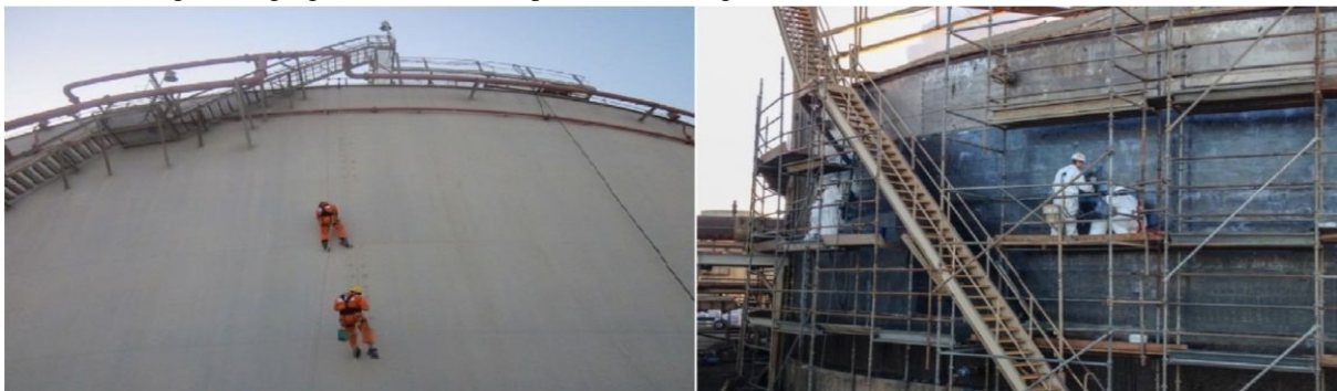
Fig. 3 Conventional Inspection Procedure [18]
