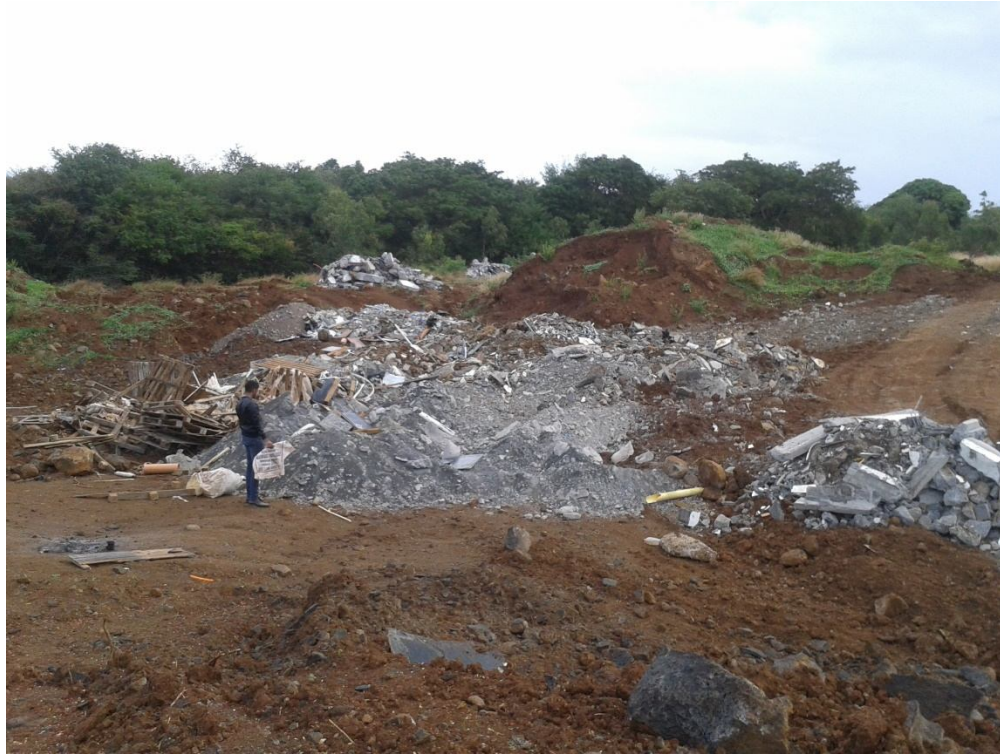
Fig. 1 Land fills deposit of C&D waste materials
