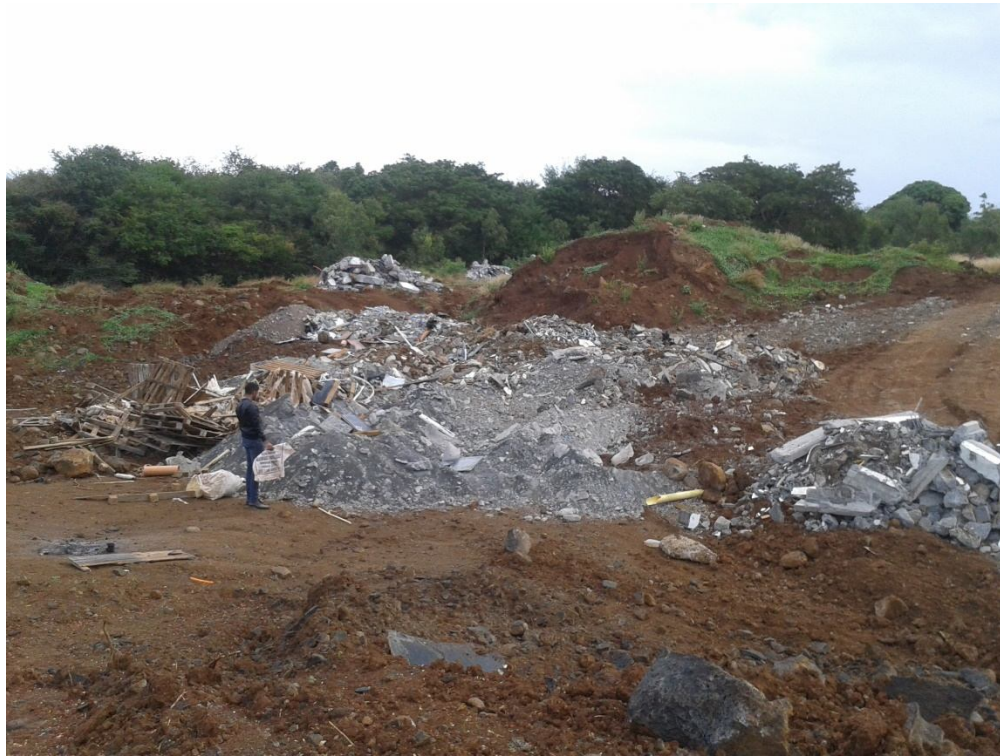
Fig. 1 Land fills deposit of C&D waste materials
