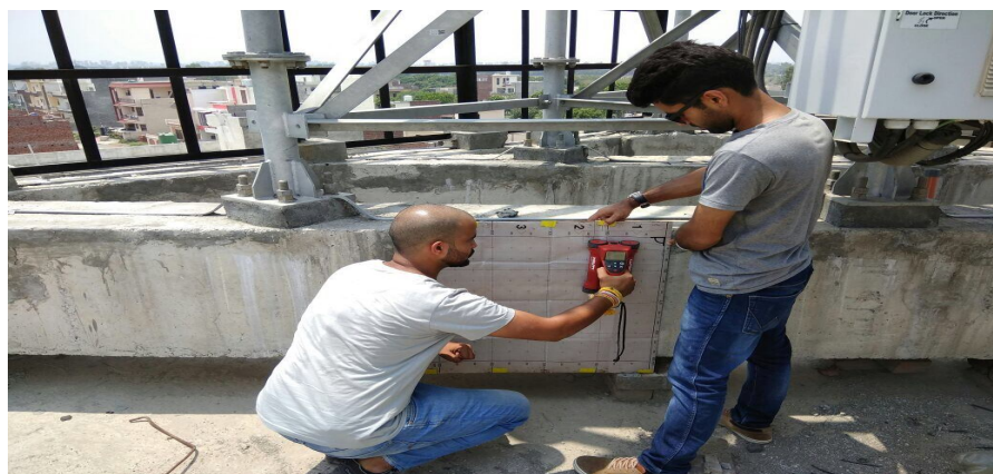
Figure 6 Conducting Ferro scanning of Beam 4
