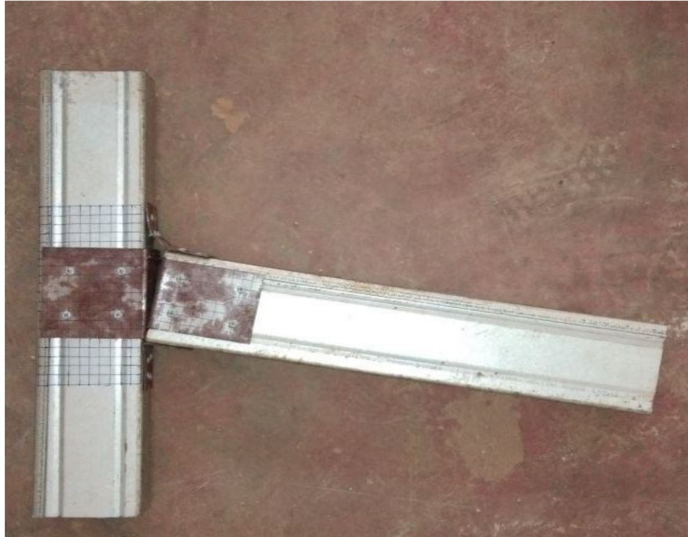
Fig. 8 Tension weld failure of beam-column connector and distortion of angle plate in Experimental Model.
