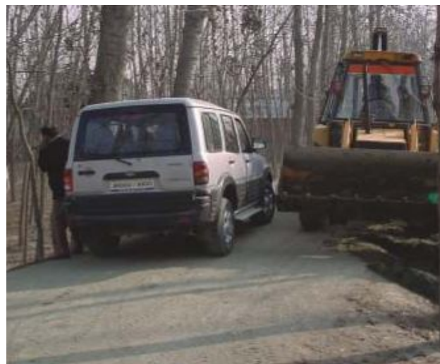
Figure 3 Laying down the road in Nagaland (Hilly Area) connecting to village.
