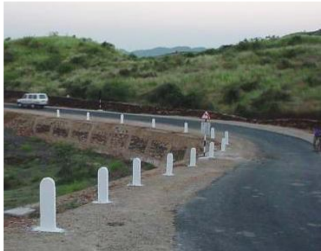
Figure 2 /Completed project under Pradhan Mantri Gram Sadak Yojna
