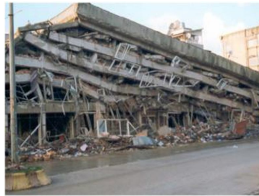
Fig. 2.4 Strong beam weak column failure (Turkey).
