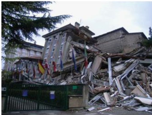
Fig. 2.2. Collapse of hotel (Italy).
