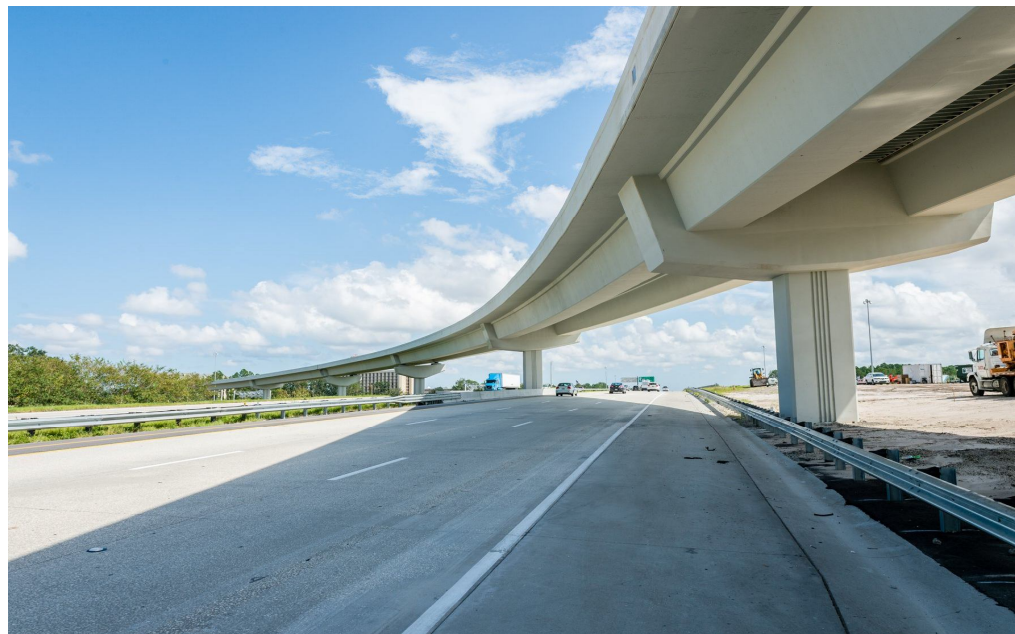
Fig-1: Girder Bridge
