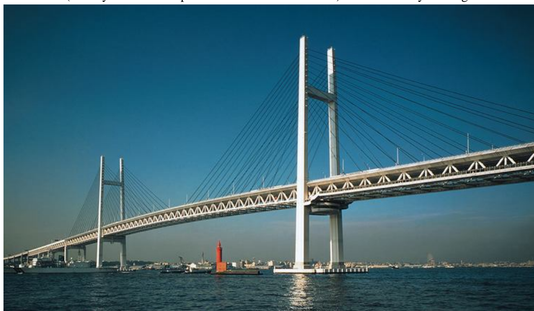
Fig-2: Cable stayed Bridge
