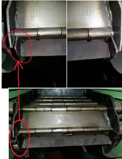
Fig. 10 Side Wing Gap
