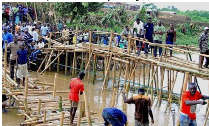
Fig. 2: showing Apete Pedestal Bridge under construction
