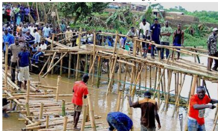
Fig. 2: showing Apete Pedestal Bridge under construction
