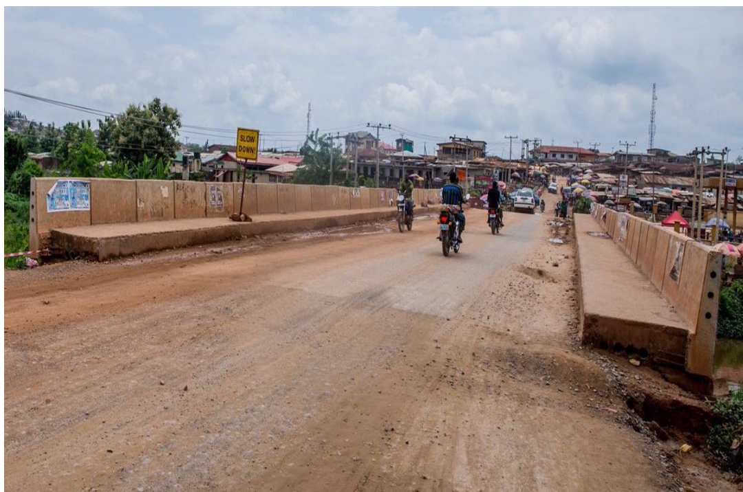
Fig. 5: Apete Newly and enlarged bridge constructed by the State Government.
