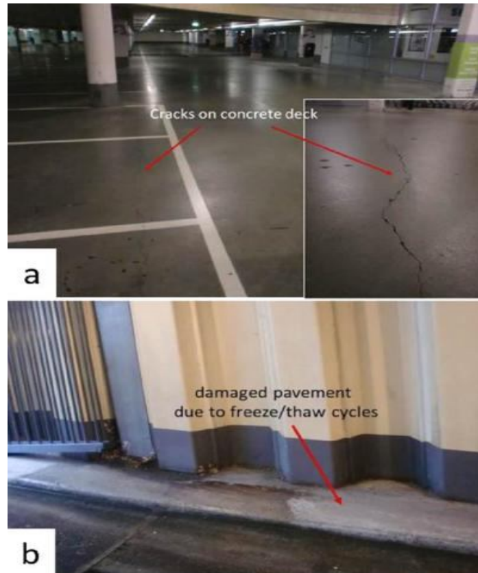
Figure 2.4 Test location for the application of the bacteria-based repair system.
