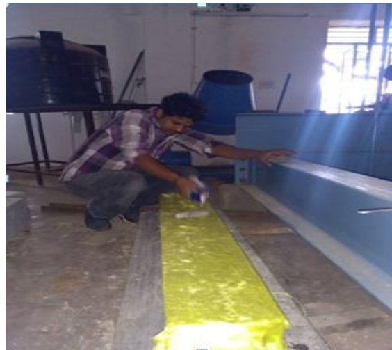
Fig 4: Application of Epoxy and Aramid fibre
