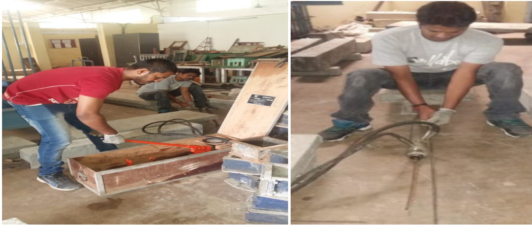
Figure.3. Post-tensioning of beams
