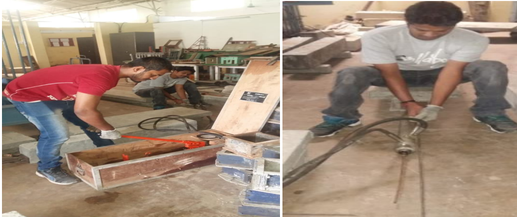
Figure.3. Post-tensioning of beams
