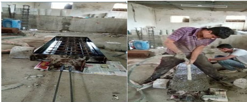
Fig 2:- Casting of Post Tensioned T- Beams
