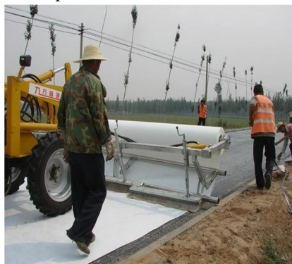
Fig. 1. Laying of Geotextile
