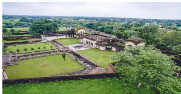
Fig.1 Aerial view of Chaman Mahal
