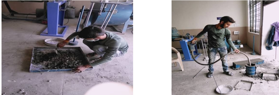
Image 1 mixing of concrete
