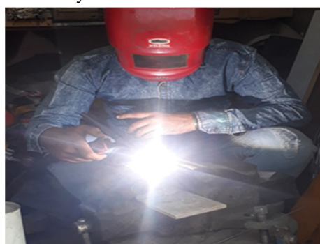
Figure 6: Welding of Plates
