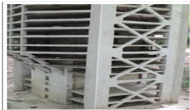
Fig.2 Provision diagonal bracing
