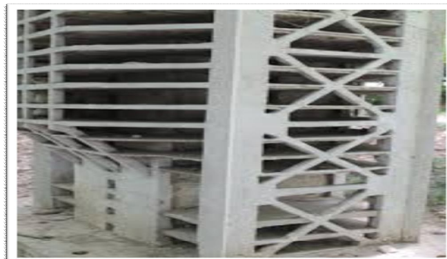
Fig.2 Provision diagonal bracing
