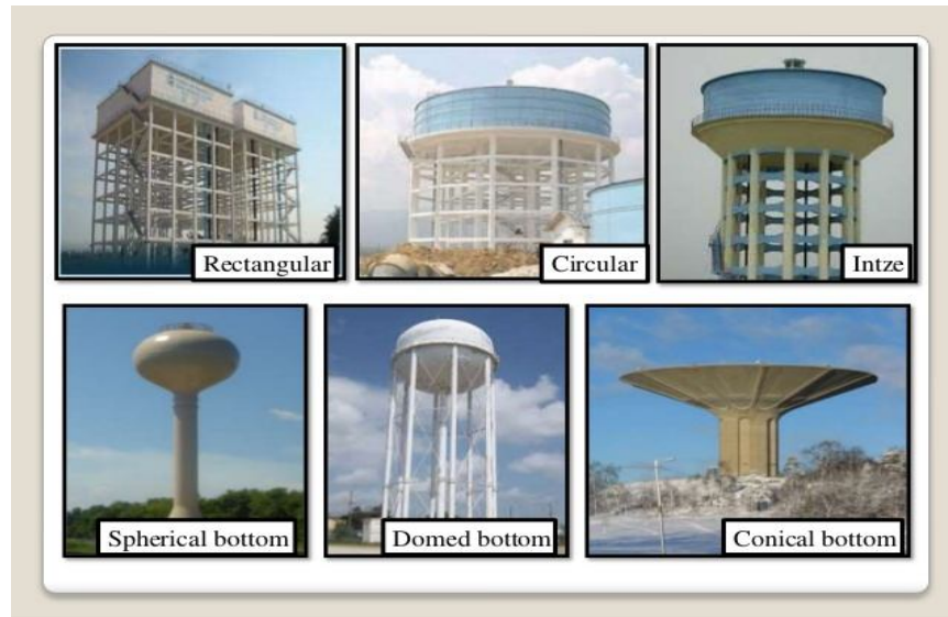
Fig. 1 Types of water-tank
